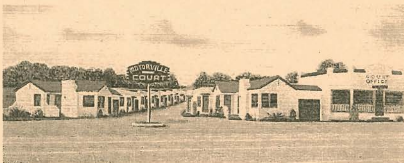
The Motorville Motel in its heyday (circa 1930) – Thanks to Michael Rocchetta and the Colma Museum. The motel, 7500 Mission St., is closed and soon to be demolished.
