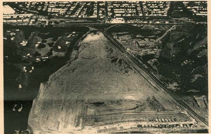
1949, Westlake after grading
