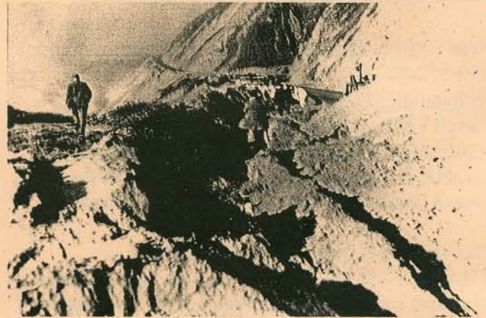
Fissures and landslides on Coast Highway, 1957 earthquake (Michael Rocchetta scanned and enhanced the photo)
